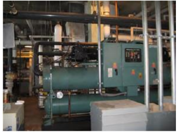
Above: York Chiller
